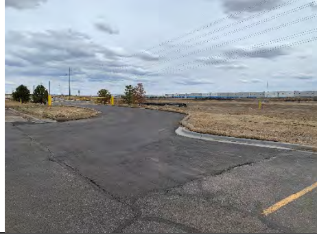
Fire Lane Improvements
