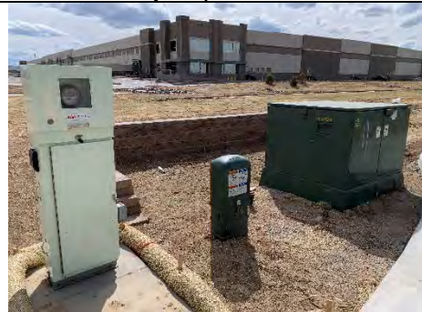
Retaining Wall Improvements
