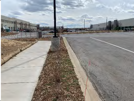
Drive into ACC Site (West Side)
