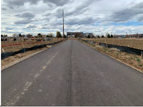
Fire Lane Improvements
