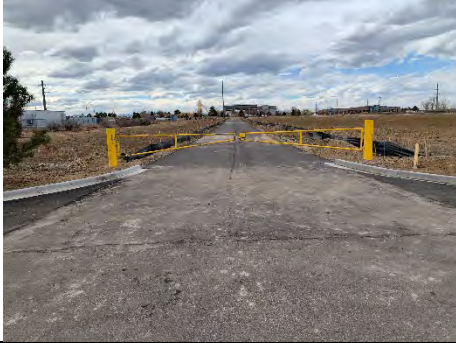
Fire Lane Improvements
